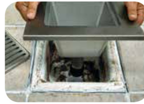
Insert stainless steel liner
